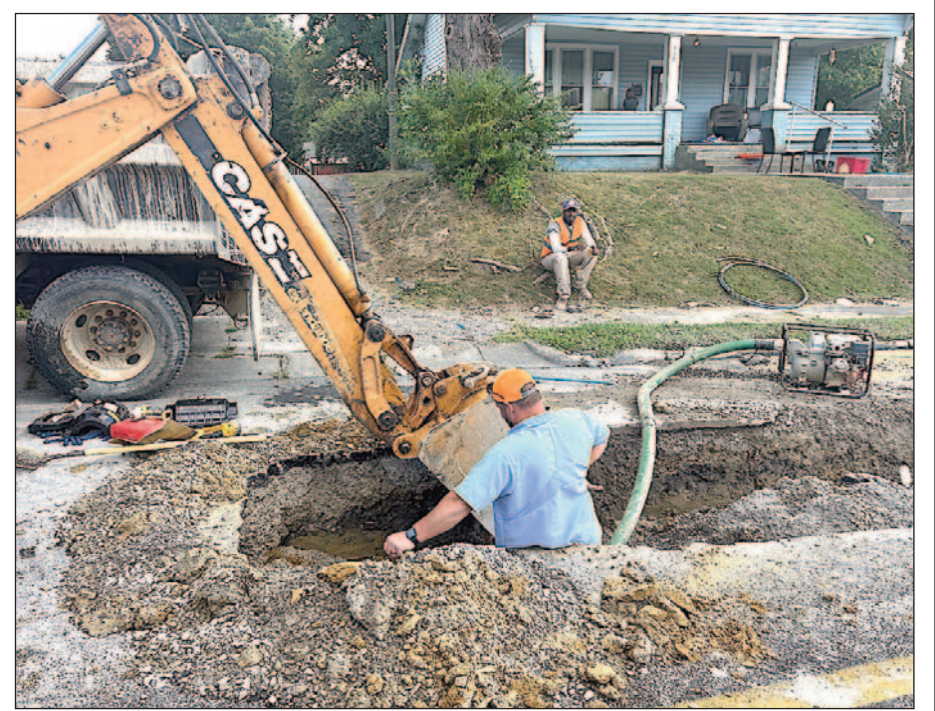
City of Marion crews have been locating and repairing water line leaks, which has taken on greater importance as the town continues to suffer from its more than three-year-old water crisis. Pictured above is City Maintenance Supervisor Greg Tabor working to repair a leak that began oozing up from beneath West Belleville Street. Tabor said a company hired to help locate leaks has found 18. He characterized them as “small leaks” that are within the city’s ability to repair, so no further contracting may be necessary. At the August Marion City Council meeting, it was noted that Marion’s current water loss is just above 25 percent. During the early stages of the crisis, those losses were approaching 50 percent, then were reduced to around 18 percent. However, recent conditions have been favorable for water line breaks, keeping the city maintenance crew busy.
